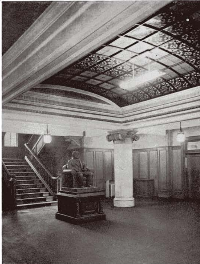
General view of the assembly hall of Japan Medical Association Building (the central figure is late Dr. S. Kitazato)
